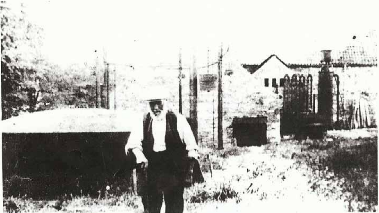
Plate IV Branston barn. The gas works with equipment in situ , 1920s. Catherine M. Wilson.
